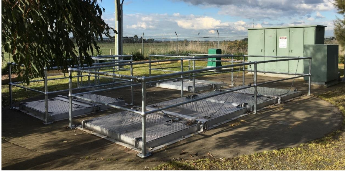
Figure 7: Example of external aluminium covers with permanent guard rails ( Note : a ground level standing area in front of the ladder inside the guardrail area has not been provided in this example but shall be provided if practical. Swing gates to enable worker entry inside the guard rail area is also required. Refer Figure 1)
