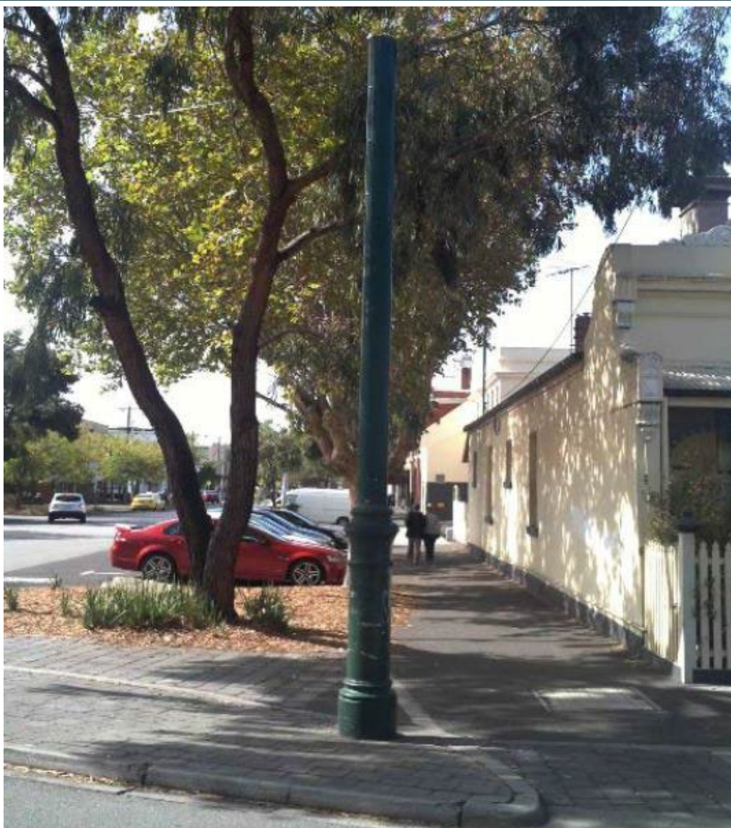
Figure 13: Sewer vent shaft
